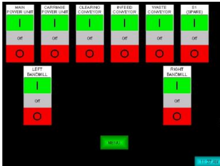
Motor Control Screen
